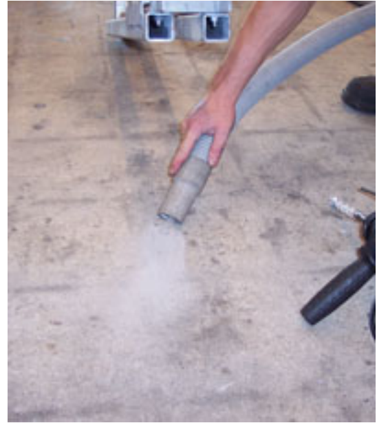
4. Vacuum the concrete dust.
