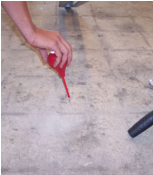
5. Or, use a blow-out bulb or compressed air to clean the dust from the holes.
